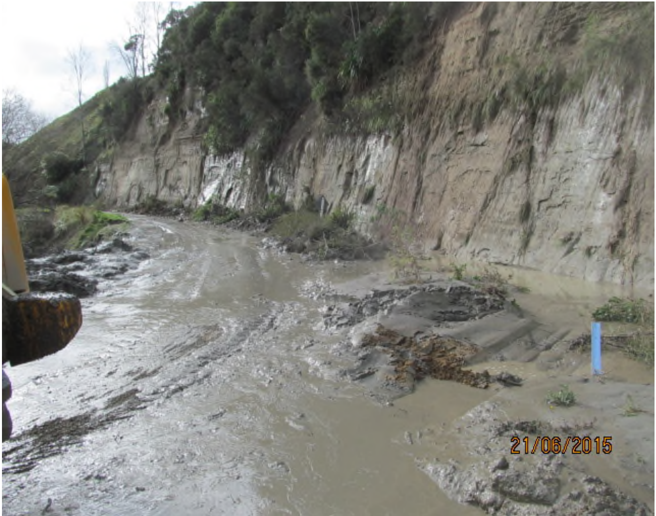
Turakina Valley Road under flood waters
