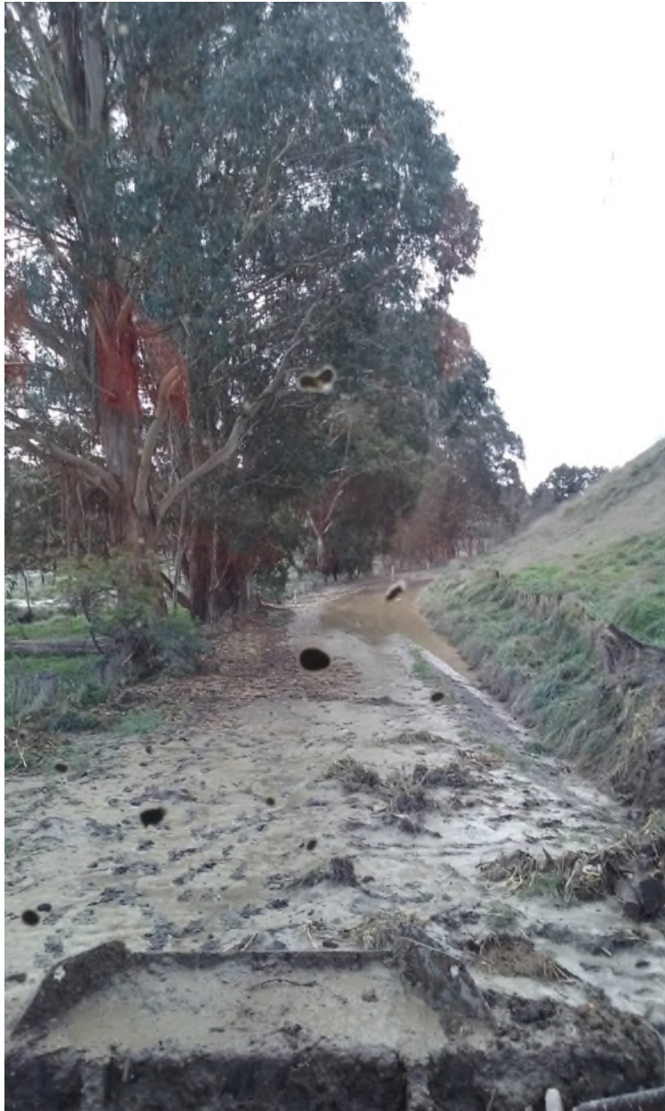
Okirae Road – impact of storm event, 20-21 June 2015
