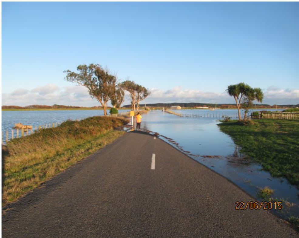
Parewanui Road, Scotts Ferry, following the June 2015 storm
