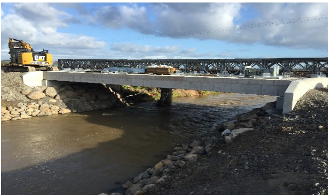
Rata Bridge replacement
