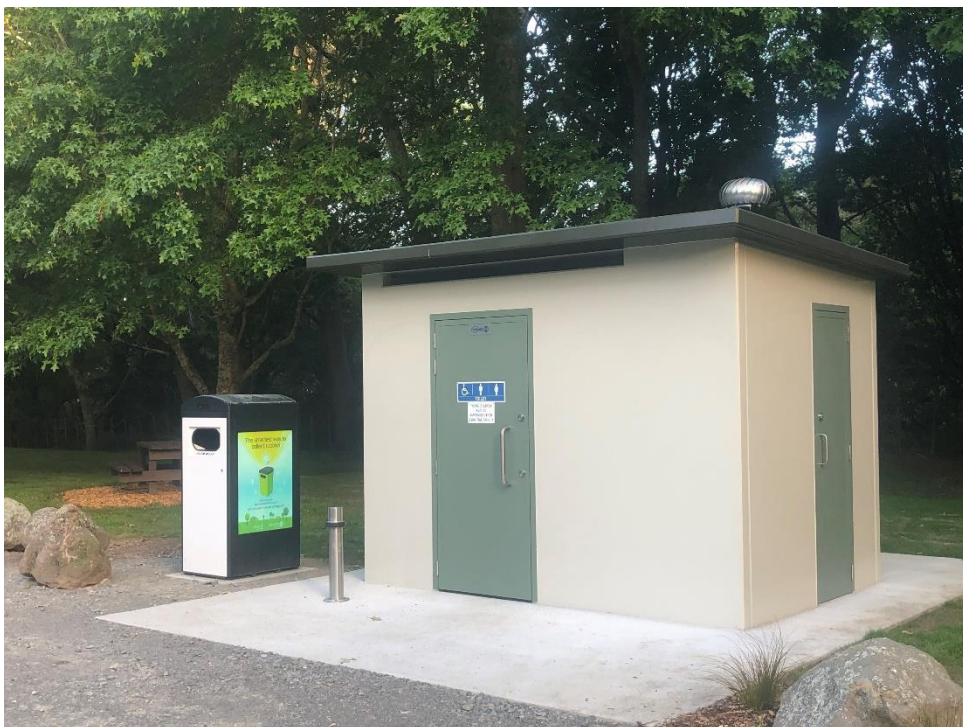
Image: Installation of Toilets - Hunterville – December 2018
