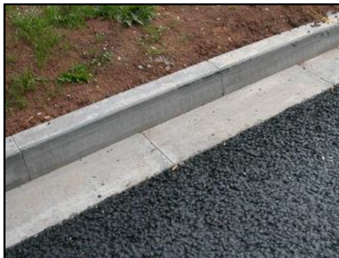
Figure 36: Standard Kerb and Channel
