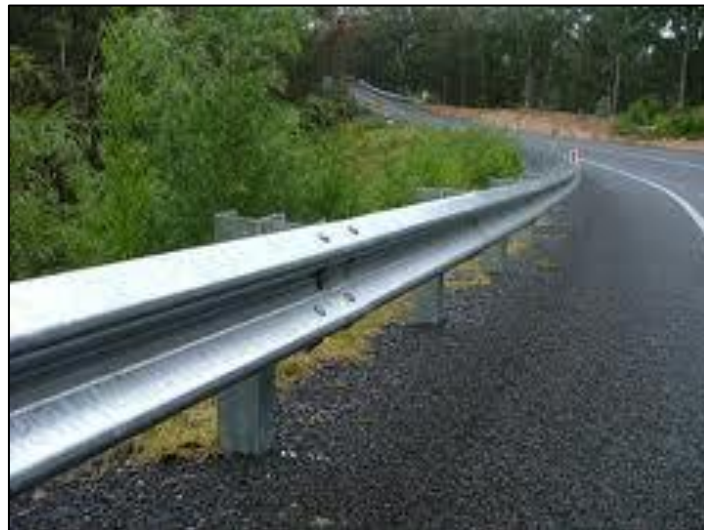
Figure 62: Armco Guard Rail
