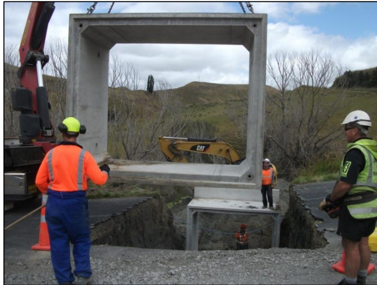
Figure 67: Stock Underpass Installation
