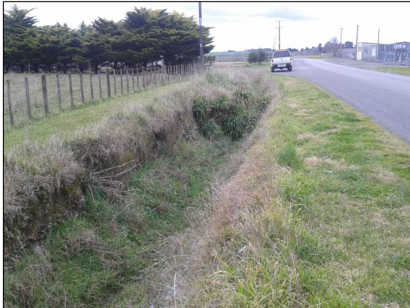
Figure 41: Deep Surface Water Channel (Watson St, Bulls)
