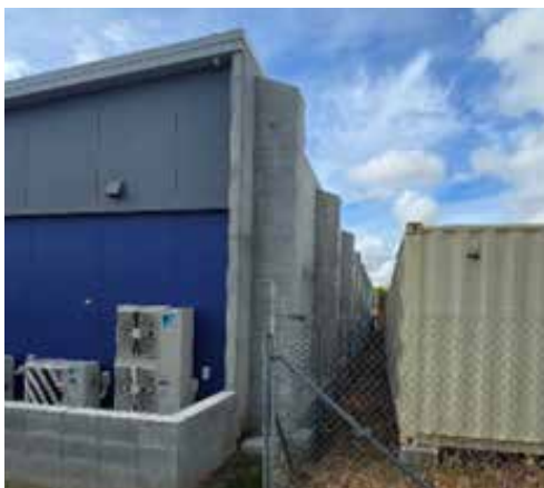
Building with concrete back wall along property boundary.
