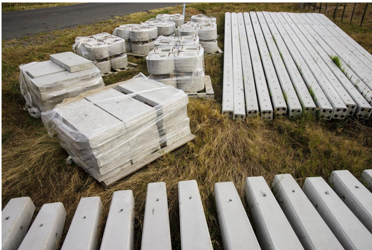
Figure 2: Power pole stockpile in preparation for upgrading an existing line. The existing power supply network in the Rangitikei District is inadequate to enable even mid-range irrigation. New irrigators are required to either fund upgrades to the existing network or install diesel generators.
