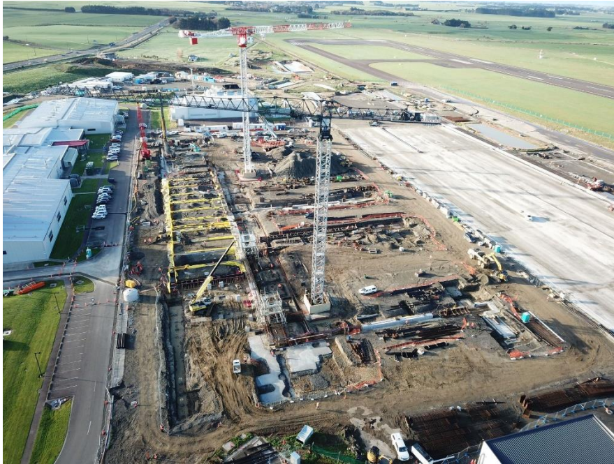
Figure 3.2: Construction of Base Ohakea.
