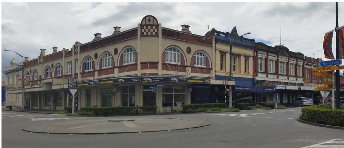
Cobbler/Davenport/Abraham & Williams buildings Broadway, Marton
