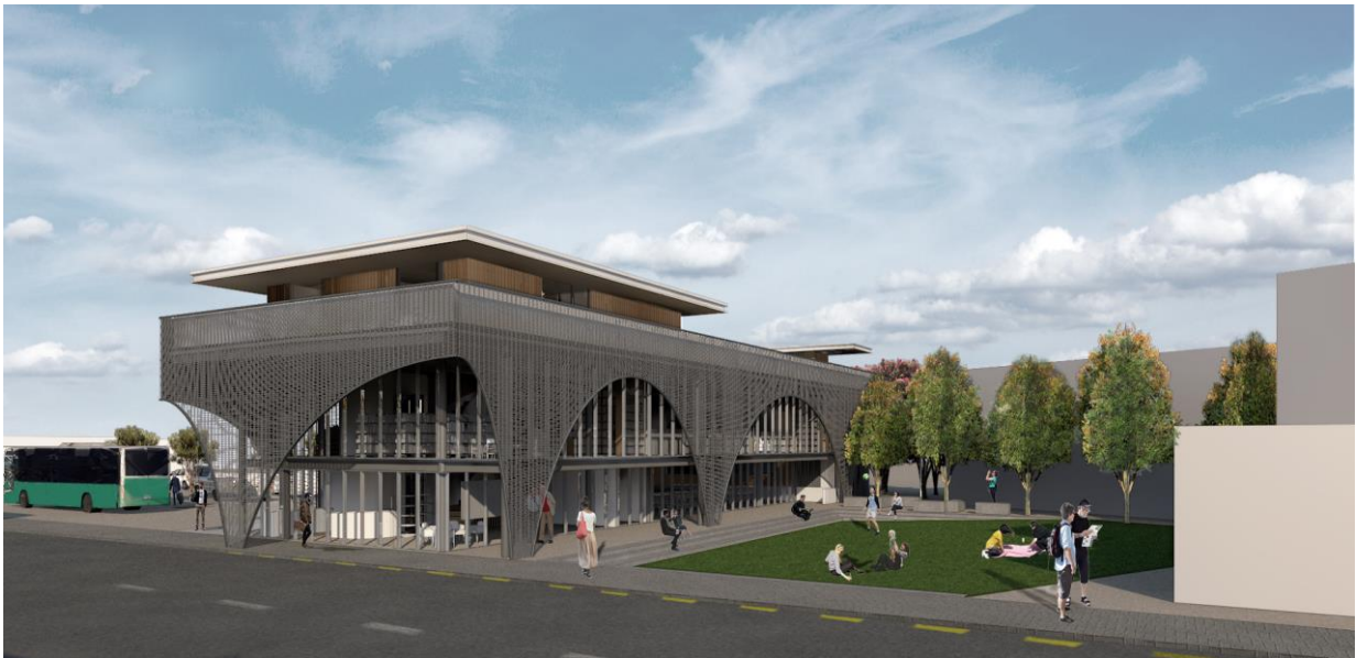
Multi-purpose Community Centre, Criterion Street, Bulls (under construction)
