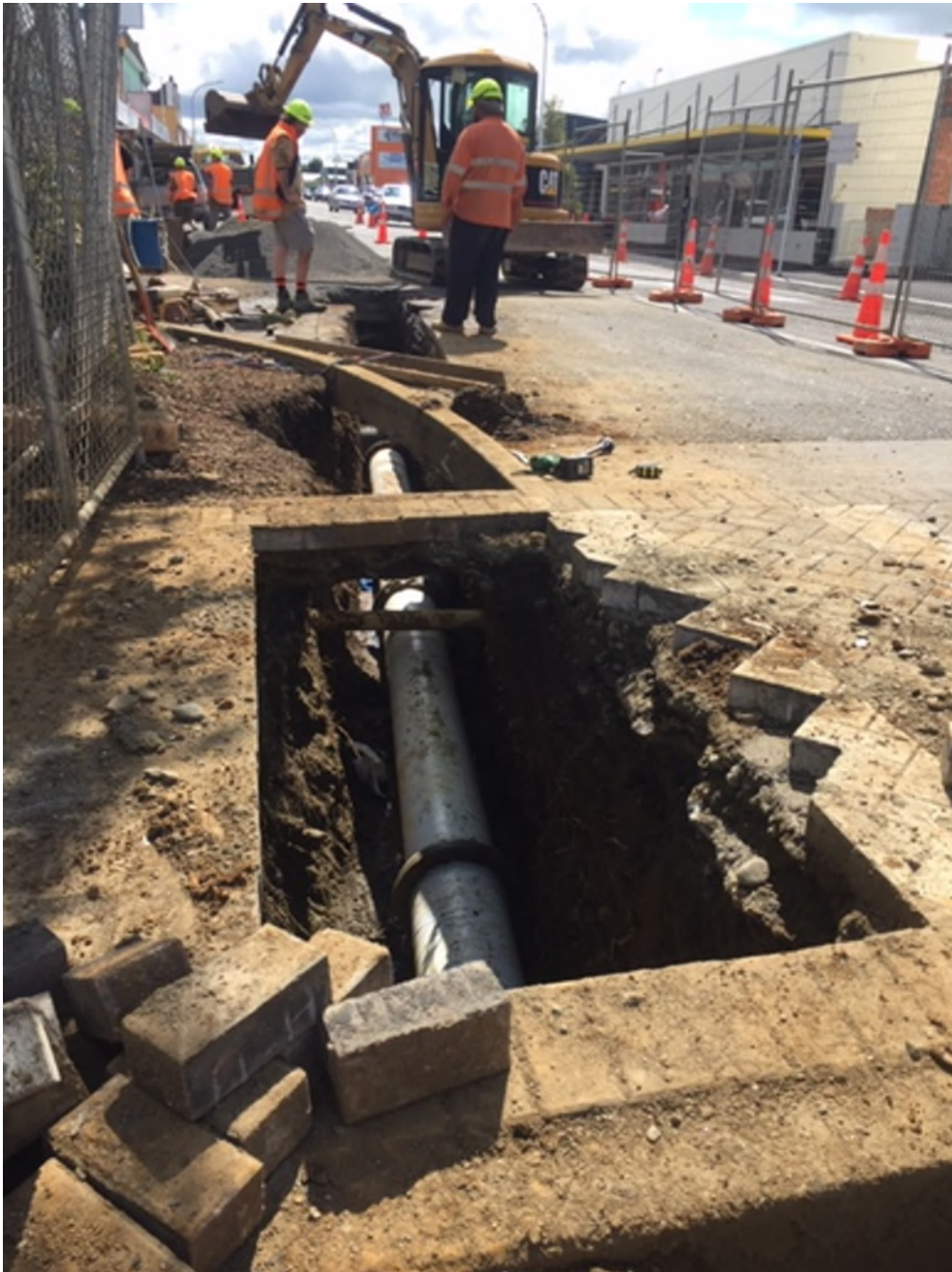
Stormwater replacement, Broadway, Marton
