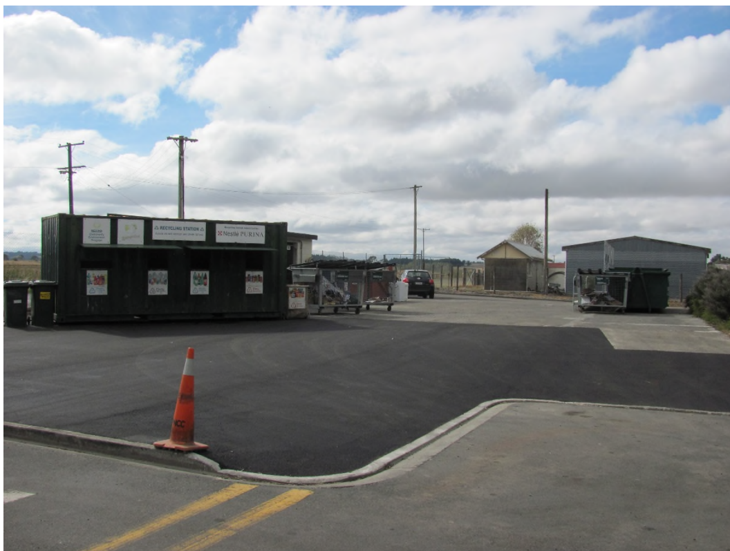
Bulls Waste Transfer Station
