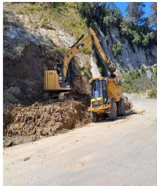
Cover photo credit: Stewart Bird, Supervisor Location: Papanui Junction (Digger Crew)
