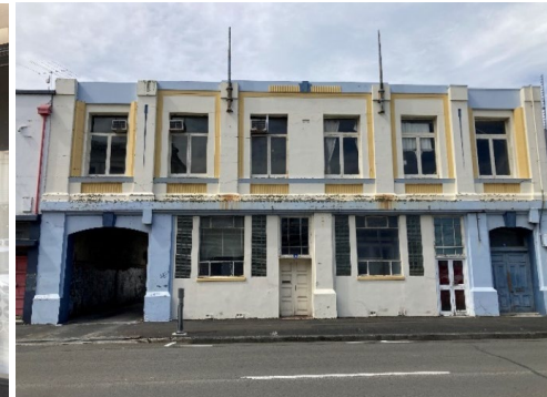
Deteriorating building. Lowe St
