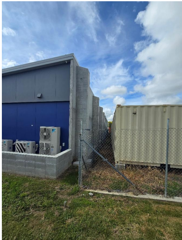
Building with concrete back wall along property boundary.
