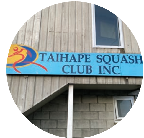
Figure 19 - Club entrance located off Kokako Street.
