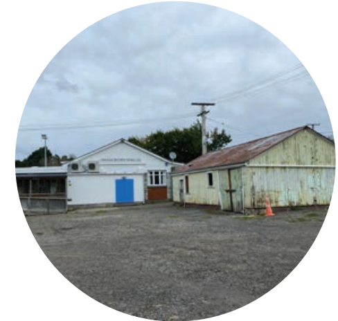
Figure 2 - Entrance point alongside Utiku Old Boys.
