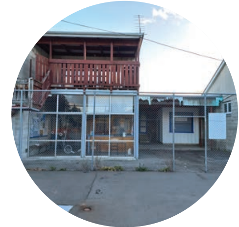
Figure 11 - Netball access, toilet and storage.
