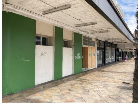
Masonic Hotel frontage. Gladstone Rd
