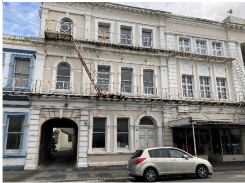
Masonic Hotel decaying façade. Lowe St
