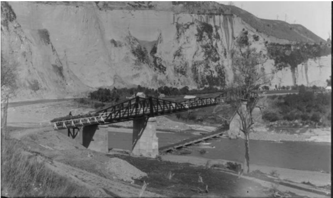
Figure 20: Completed cantilever bridge with low-level bridge beneath
