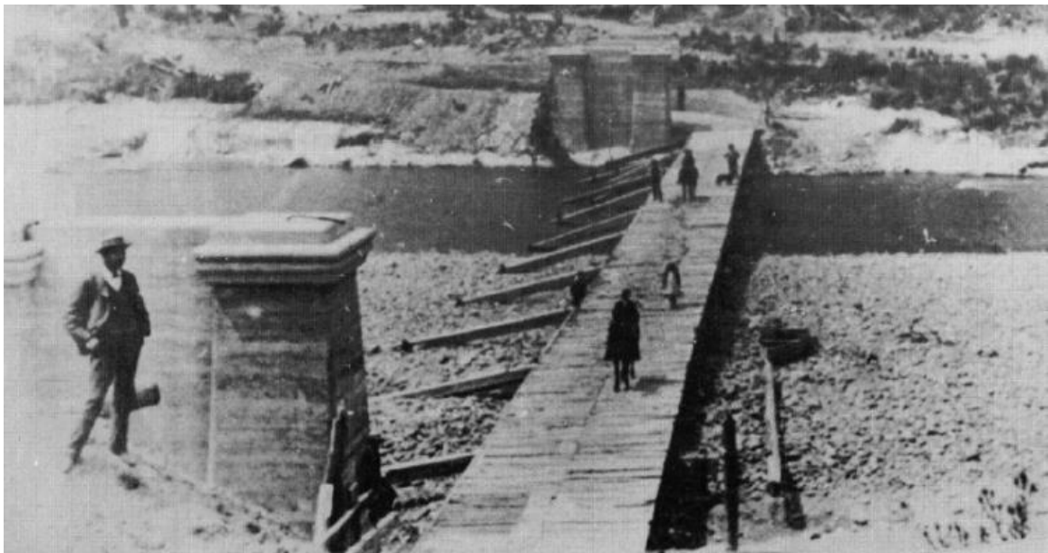
Figure 16: Low-level bridge c.1897 with concrete piers for permanent bridge on upstream side looking east (reproduced from Mangaveka and District's First 100 Years)
