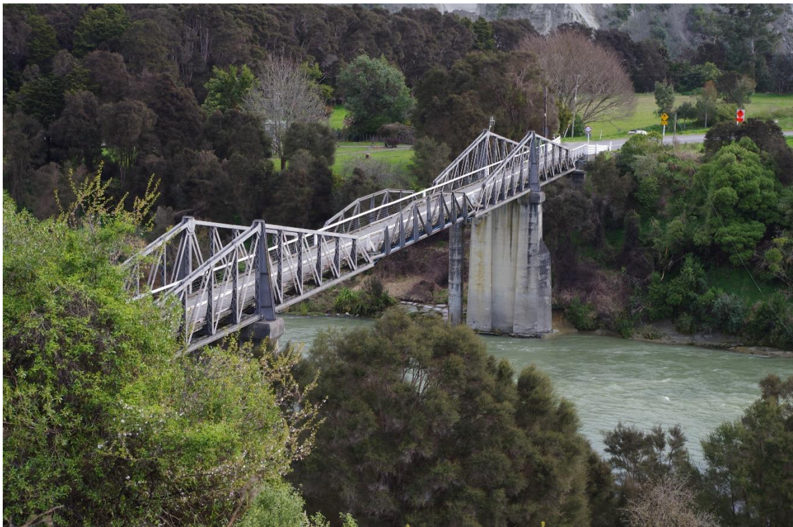
Figure 35: Mangaweka bridge viewed from eastern side
