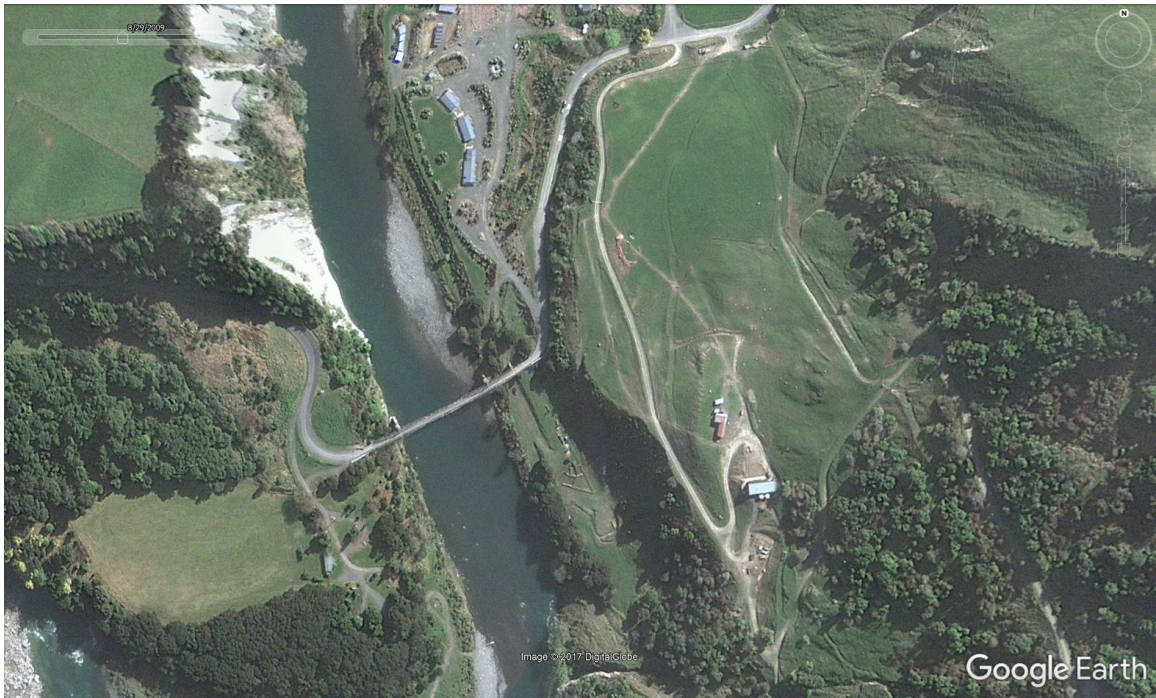
Figure 3: Google Earth imagery dated August 2009 showing the Mangaweka bridge and approaches
