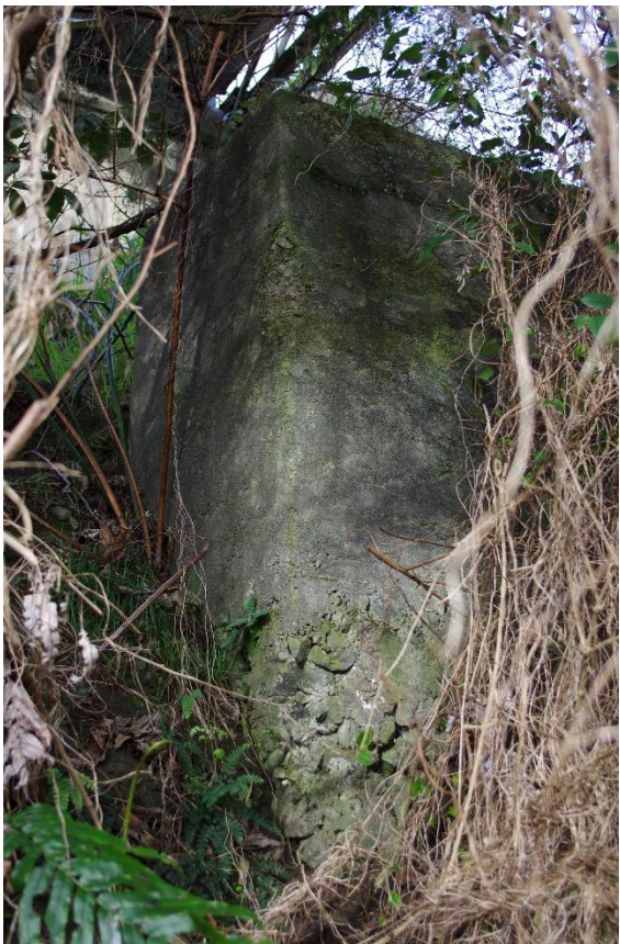
Figure 32: 1897 abutment on eastern side, viewed from below
