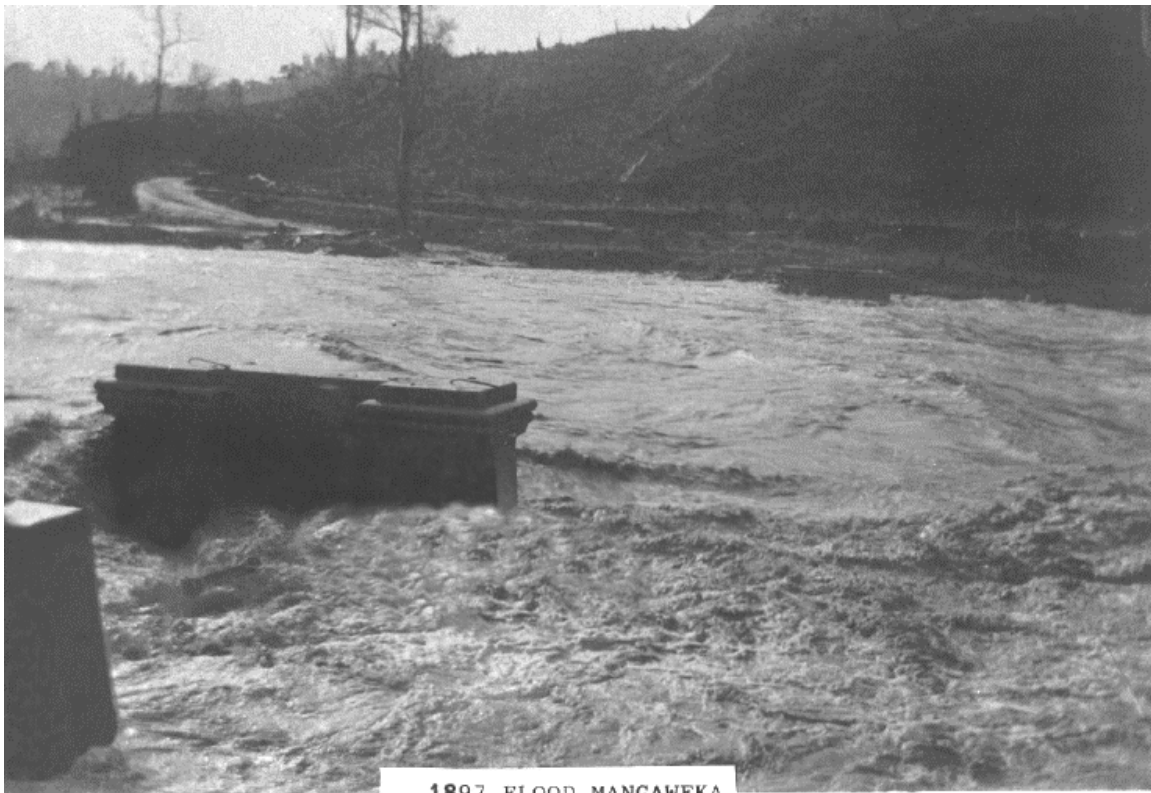
Figure 17: Photo showing the height of 1897 flooding relative to the concrete piers (reproduced from Burr 2017)
