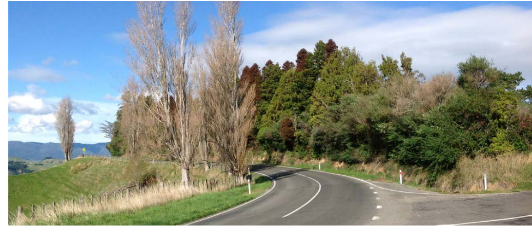
View from Rangiwahia Road looking south
